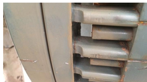
Fig. 7. Broken bars in the motor A.
